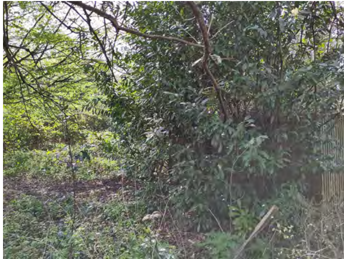
Cherry Laurel in the sub-station area
