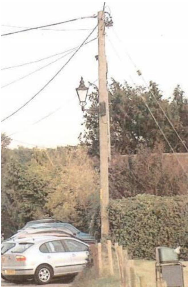
Typical overhead electricity wire with gas-type street lighting.
