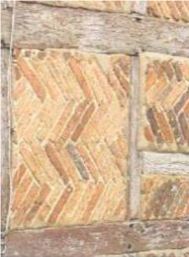
Infilling with herringbone brickwork between Tudor timber frames
